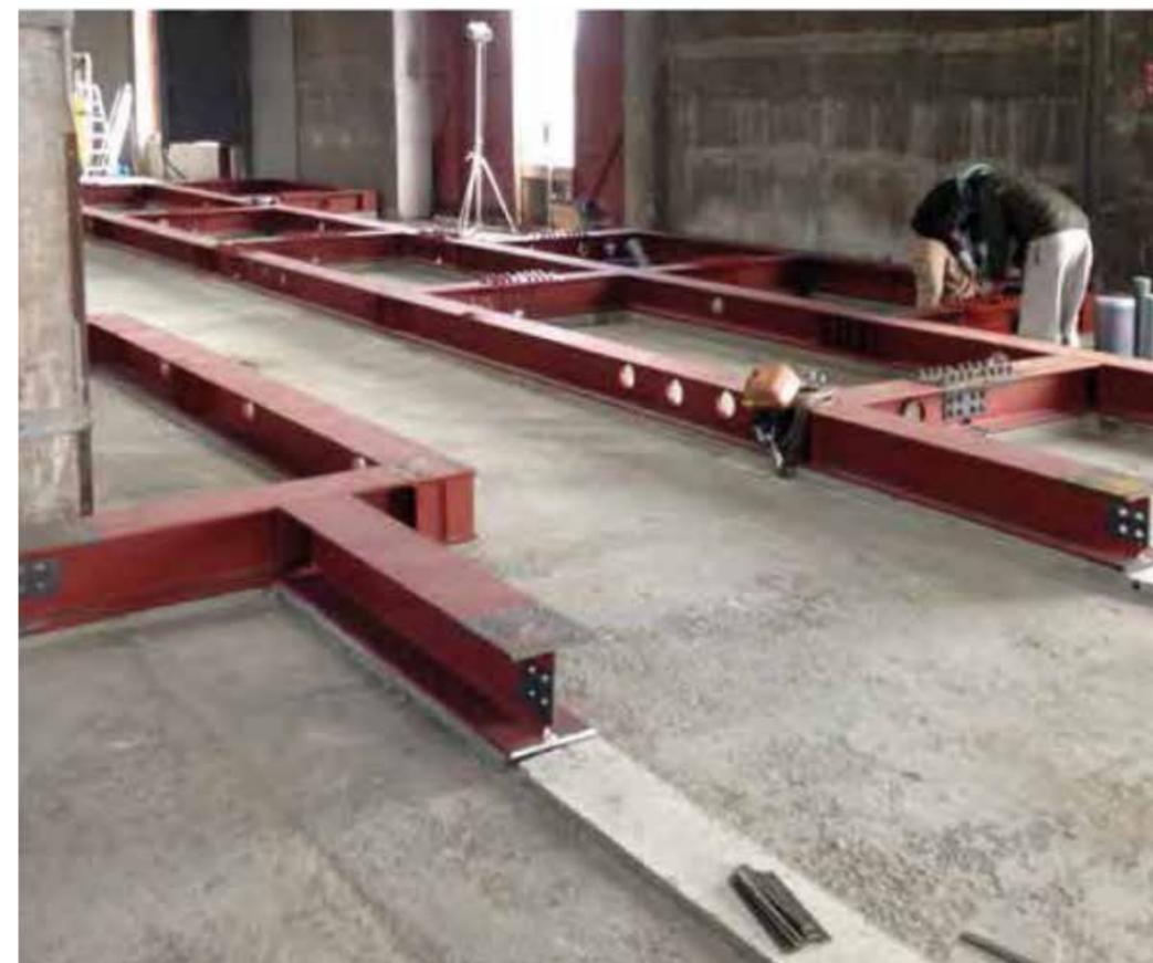
Step 1: Put steel beams on mortar. This works instead of the RC...
