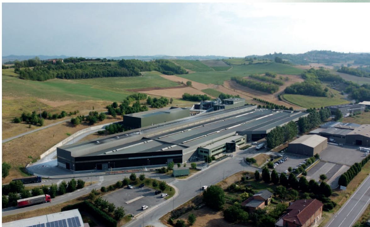
Production plant in Calliano (Asti, IT)
